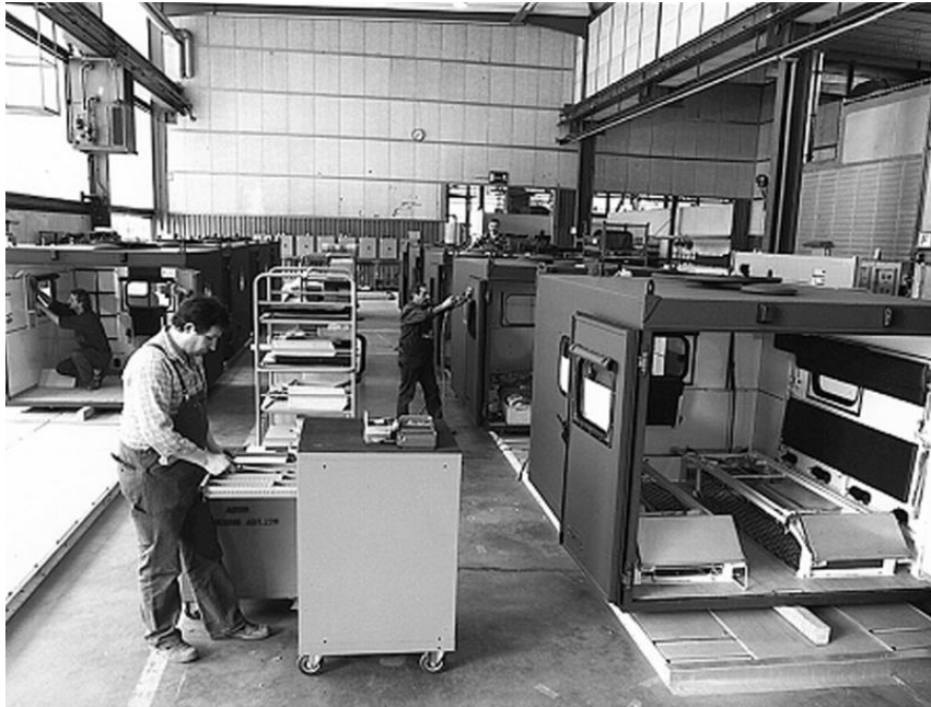
Development and production of the first Zeppelin-Shelters in the 1960s and 1970s.
